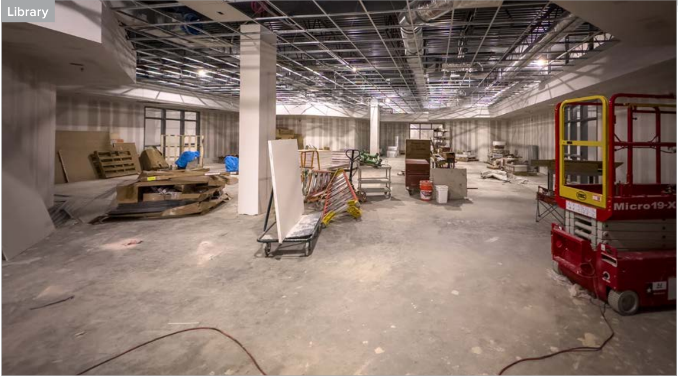
Secondary Corridor (Cafetorium/Gymnasium)
