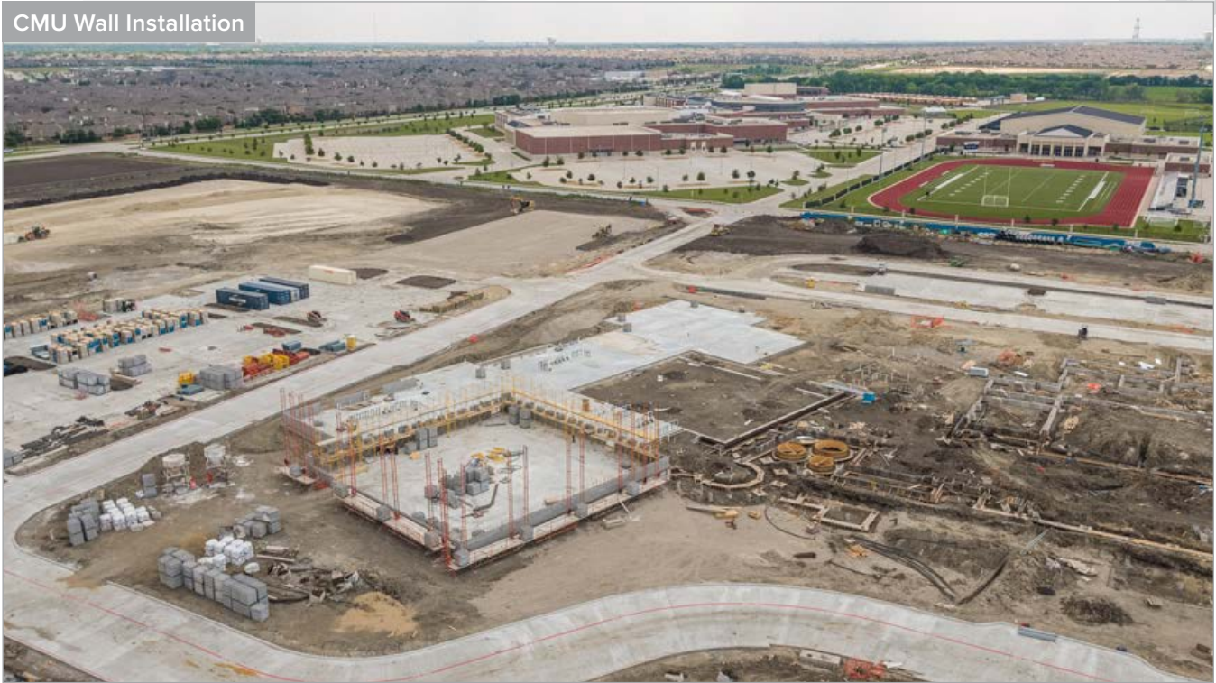
CMU Wall Installation
